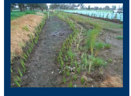
Drainage revegetation project.
