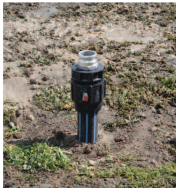
Newly installed hydrant for effluent distribution
