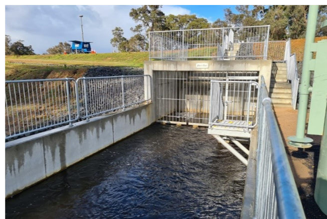
The completed penstocks
