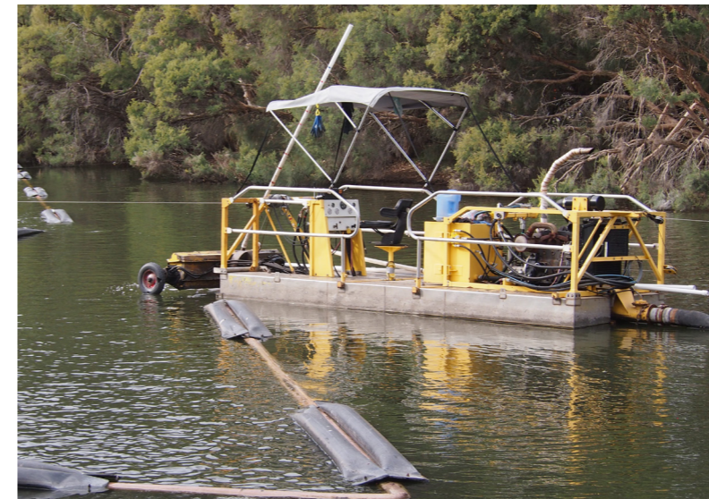
Micro-dredge removing sediments in the Lower Vasse River
