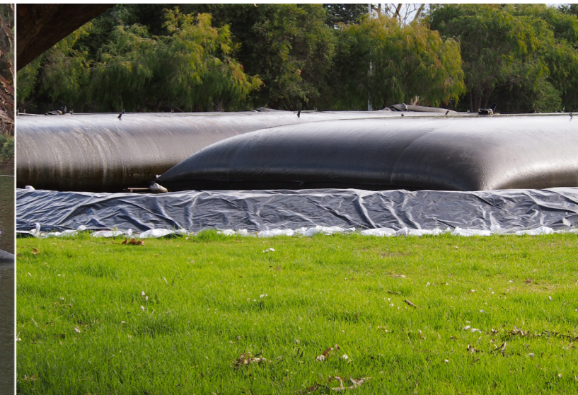
Dewatering sediments in geotextile bags
