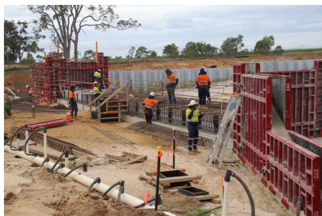
Installation of the culverts and penstock
